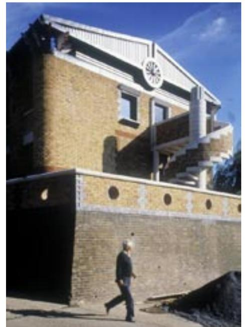
**AFTER:** Even though stripped to the steel frame, some old stock bricks on the 'blind' end wall were kept and patched into the new end. London stock brick was included in the the balustrade and spiral escape stair.
